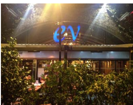
Refurbished rail arches, Isabella Street, Southwark
