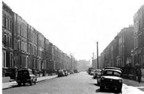
In the early 1960s Somerleyton Road retained its dignified, double-sided character. Our proposals will restore this character, but update and transform the street's programme of uses
